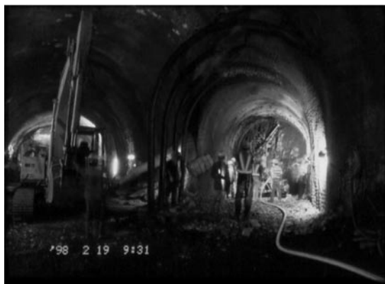
(a) Construction of Bypass Tunnel
