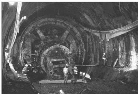
Photo 3. Dismantling of the WB TBM
